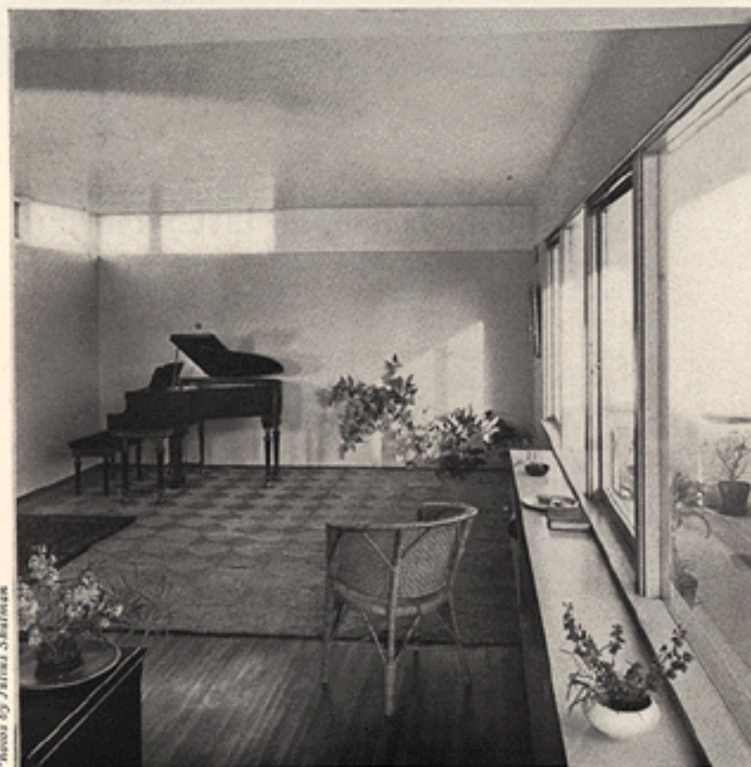
Toward the patio, the sill level of the windows is dropped to 26 in.
