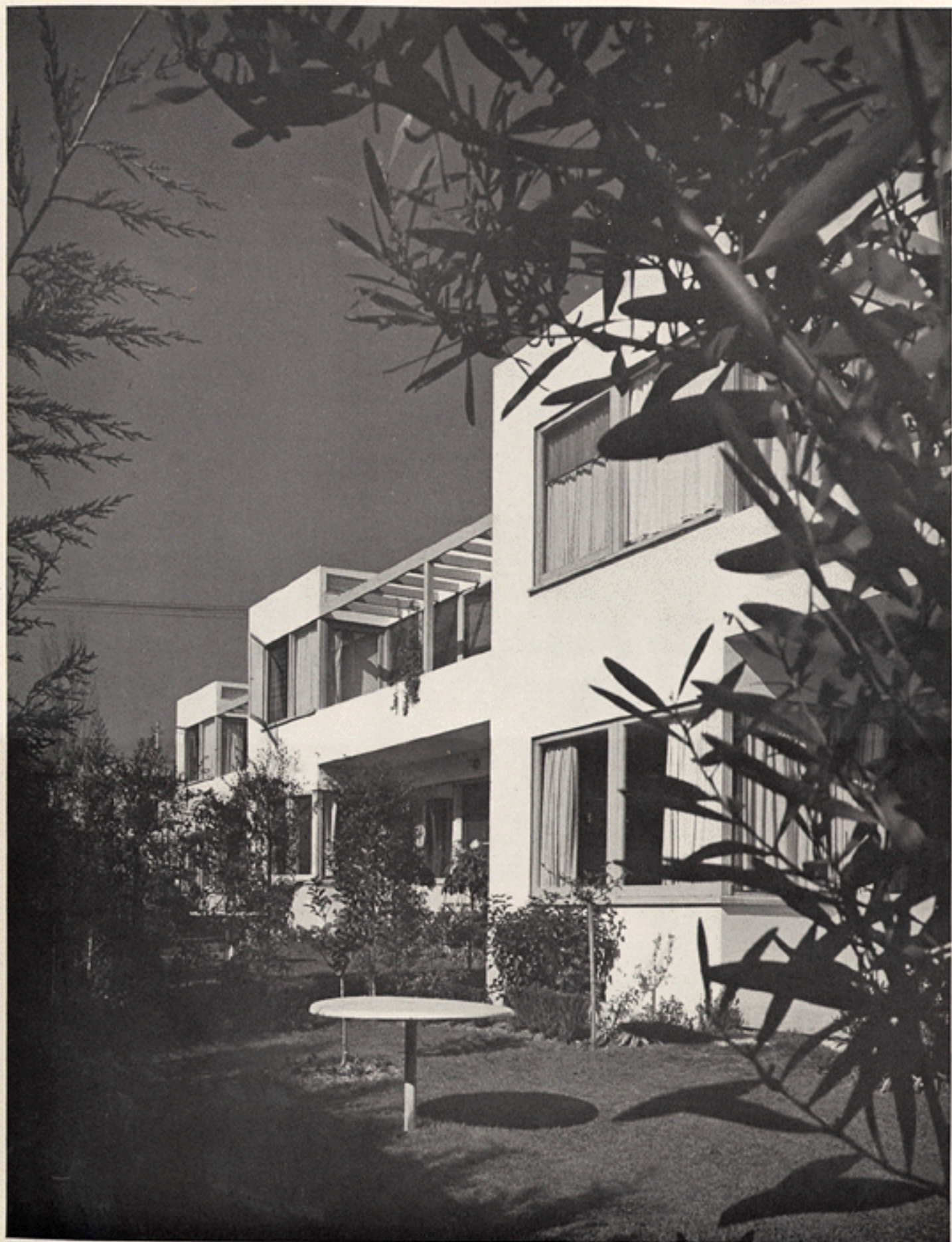
The garden front of the Dunsmuir Flats. Note how the step-back arrangement contributes to the privacy of the individual units
